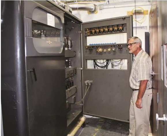
Moersdorf and his “Big Bertha” 1946 Collins 20T. It was designed for 1 kW operation and weighs in at a whopping 5,700 pounds. (That’s less than 0.2 of a watt per pound.)
