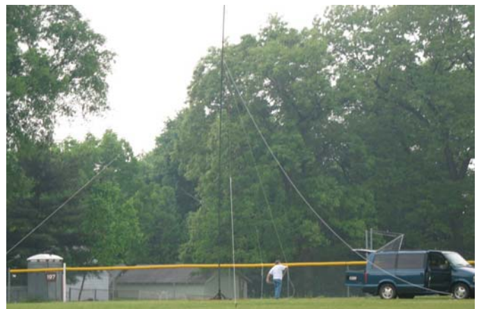
N8EQJ with the 40 meter pole up and guyed
